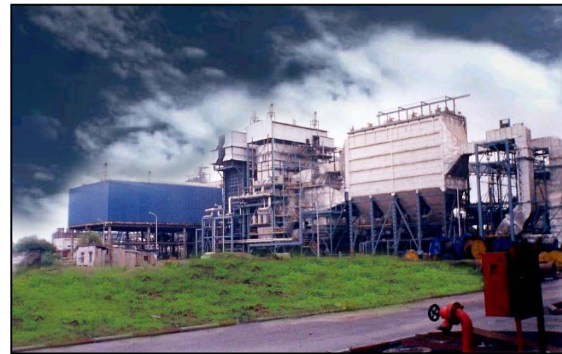
23 MW CPP-Grasim Industries, Chittorgarh (Rajasthan)
