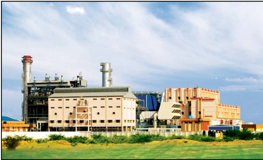
95 MW CCPP - TNEB, Ramnad, Tamil Nadu
