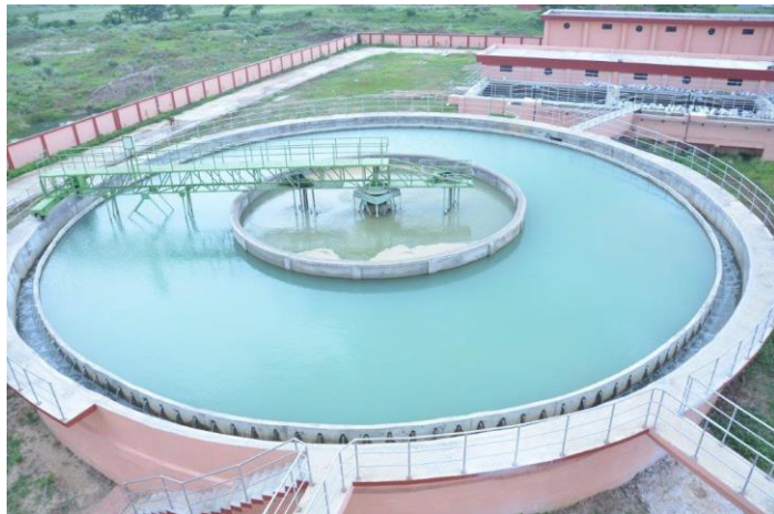
30 MLD WTP, Puri, Odisha
