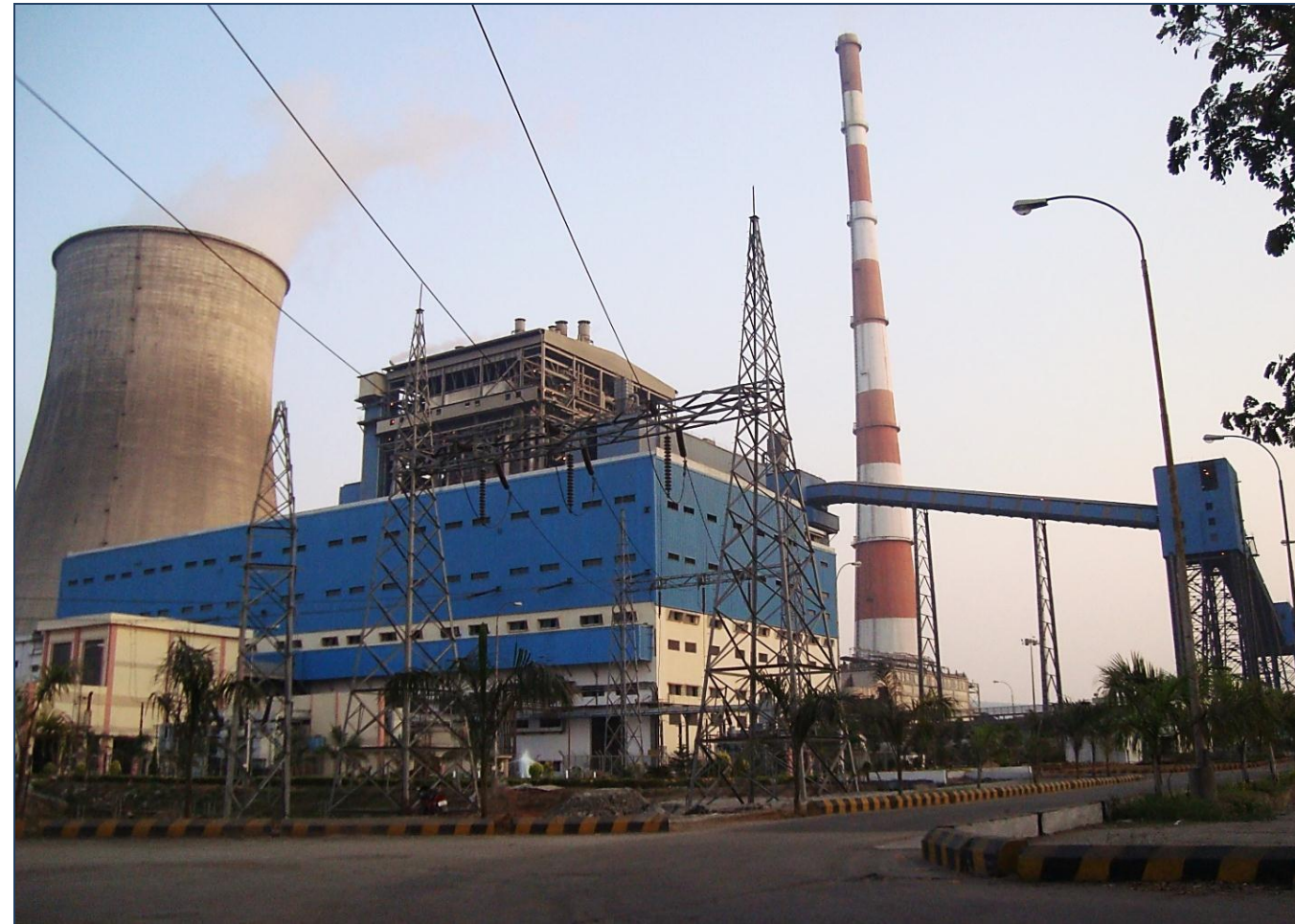
500 MW THERMAL POWER STATION - KOTHAGUEM
