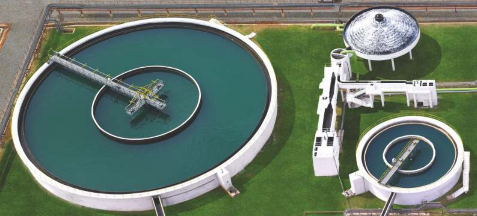
Pretreatment Plant at 500 MW KTPP, Warangal. A.P
