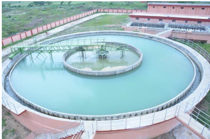
30 MLD WTP, Puri, Odisha
